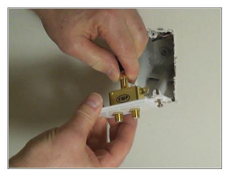
Connect the new two-way splitter plate to the coaxial cable.
