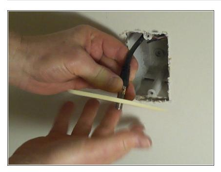
Remove the existing wall plate by unscrewing it from the coaxial cable in the wall.
