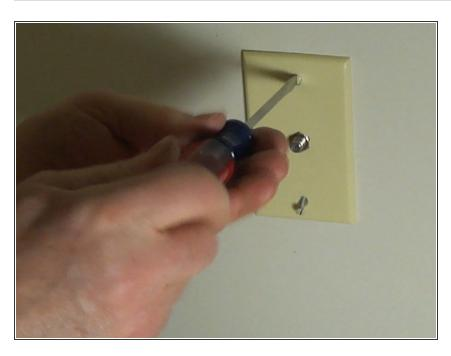
Use an appropriate screwdriver to remove the wall plate mounting screws. This wall plate used flathead screws, but yours could be Phillips.
