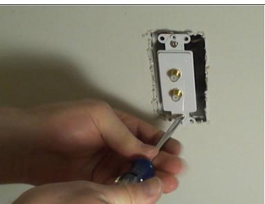
Replace the mounting screws and tighten them with the proper screwdriver.
