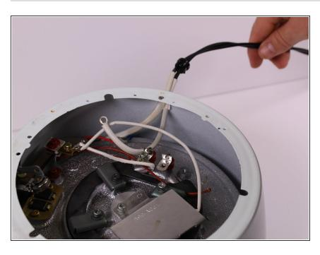
Pull the power cord through the hole, isolating the power cord from the device.
