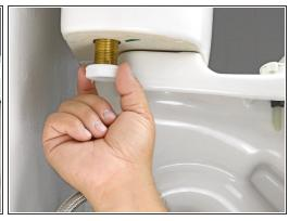
Turn the locknut counter-clockwise until it releases from the threaded shank.
