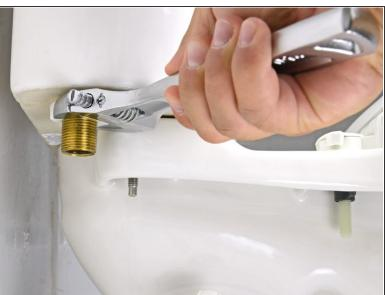
Using an adjustable wrench, turn the locknut on the threaded shank counter-clockwise until it becomes loose.
