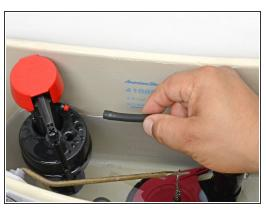
Disconnect the fill valve's rubber refill tube from the top of the overflow tube.
