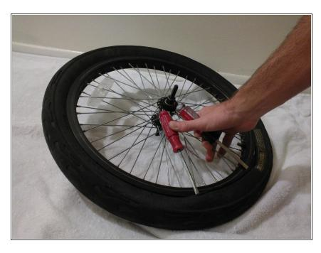
Use a second screwdriver and repeat step 3 to create a four to six inch lip where the tire overlaps the rim.
