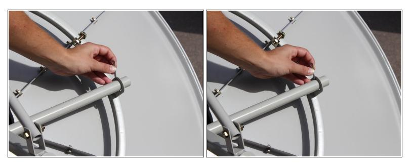
Insert a cotter pin through the holes at each end of the cross bearer.
