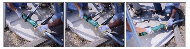
• Using two pipe wrenches, unscrew the cylinder from the riser main.
