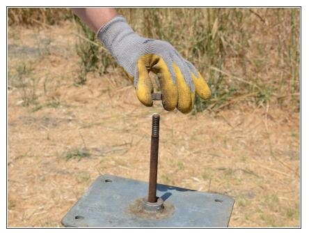
• Remove the jam nut from the top of the pump rod.
