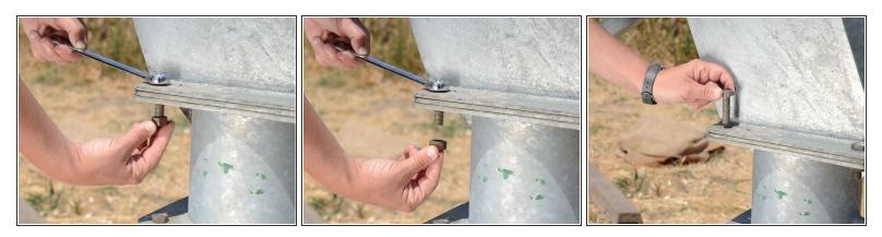
Remove the two bolts and nuts from the handle side.
