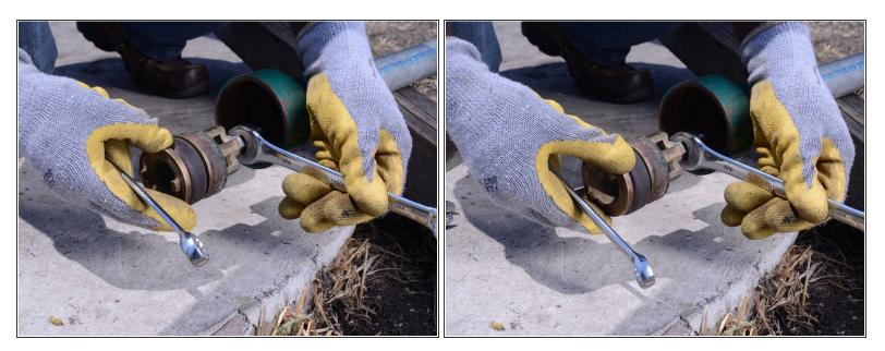
• Unscrew the valve from the pump rod.
