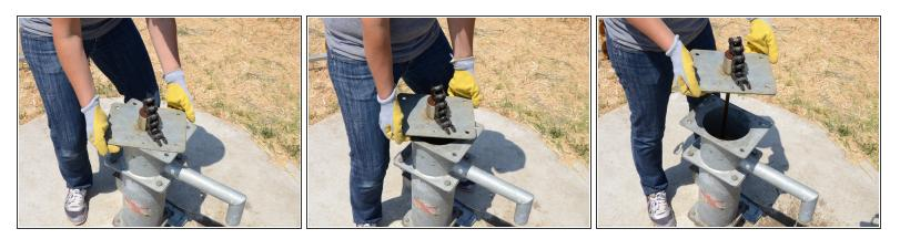
• Lift the head flange up about one foot above the tank.
