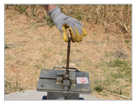
• Screw the jam nut back onto the top of the pump rod.
