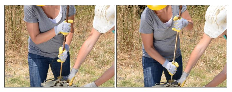
Make sure there is at least 6 inches of space between the joint and the rod clamp to allow yourself enough room to work. If necessary, continue pulling the rod out of the well before tightening the rod clamp to ensure sufficient spacing.
