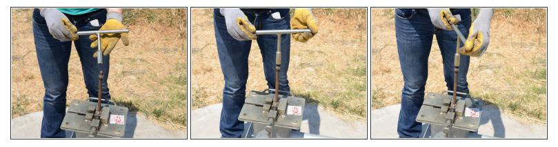
• Screw a T-handle onto the top of the pump rod. Tighten the T-handle against the jam nut.
