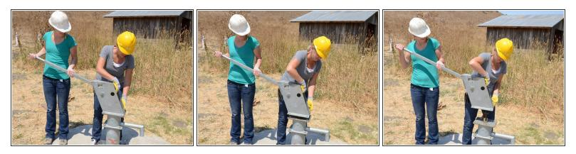
• Lift and remove the pump head from the pump.
