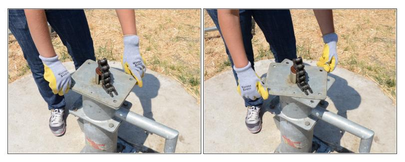
• Slightly twist the head flange, until the corners overhang the top of the tank far enough to grab.
