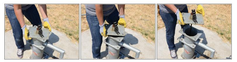
• Lift the head flange up about one foot above the tank.
