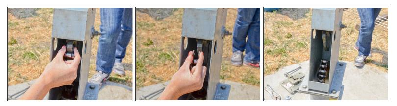
• Pull the top of the chain straight off of the pump handle.
