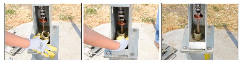
• Place the spacer collar around the pump rod below the raised chain, with the beveled side down, and the flat side facing up.
