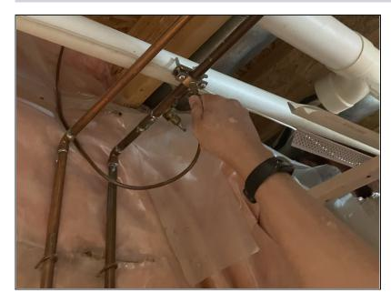
• Twist the valve to turn the water supply off for the fridge.
