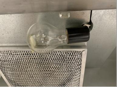
Install the new lightbulb and turn it clockwise.
