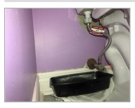
To remove any excess water from the tank. Place a container to catch the water that might drain by placing a bucket with a towel underneath the toilet to catch any water.
