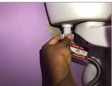
Attach the Bullock Nut to the threads on the bottom of the toilet tank and hand tighten the nut counter-clockwise.
