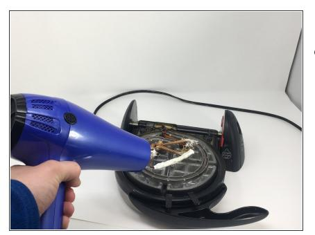
Use a hair dryer or heat gun to shrink the insulator to the shape of the new thermal fuse.
